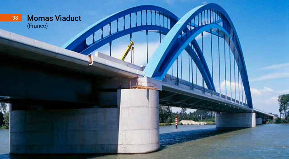
HSR viaduct on the Valence-Marseille high-speed line.
