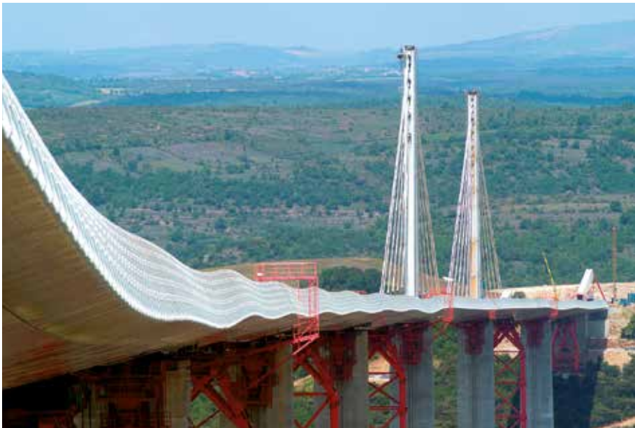
Deformed shape of deck during launching
