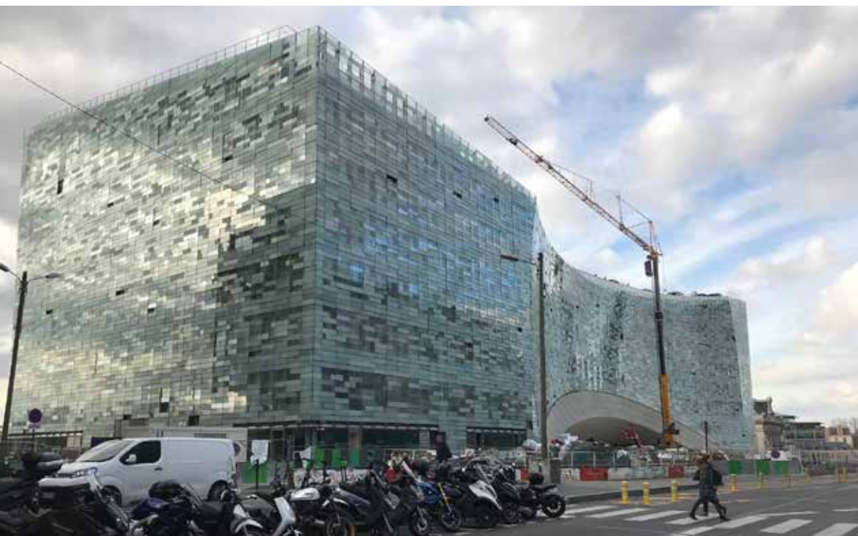
New «Le Monde» headquarters in Paris (total floor area of 23,000 m 2 )
