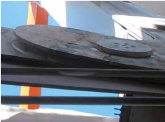
Plastification pattern in the cover plate
